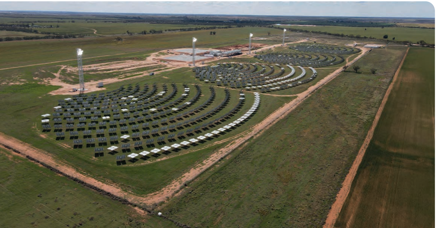
► Figure 3. Construction of the 4 MW electricity plus 3 MW/ 50 MWh storage project near Mildura, Australia, is nearing completion. Each solar field utilises nearly 300 mirrors to concentrate light onto a central receiver. (The cold and hot water pits can be seen behind the fields of mirrors.)
